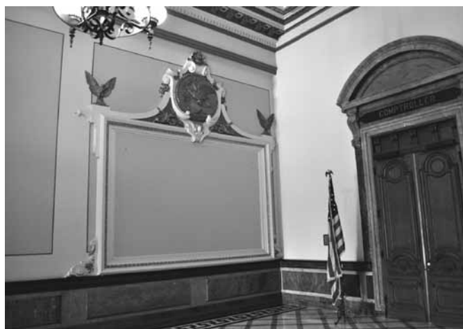
This empty frame located on the west wall of the second floor, just outside the Comptroller’s Office, used to contain a painting and a map at different times. Photo courtesy of Mark Sorensen.
