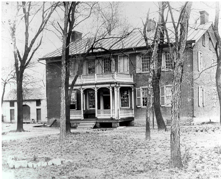
The Jarrot Mansion circa 1894. (Photo courtesy of the Illinois Historic Preservation Agency)
